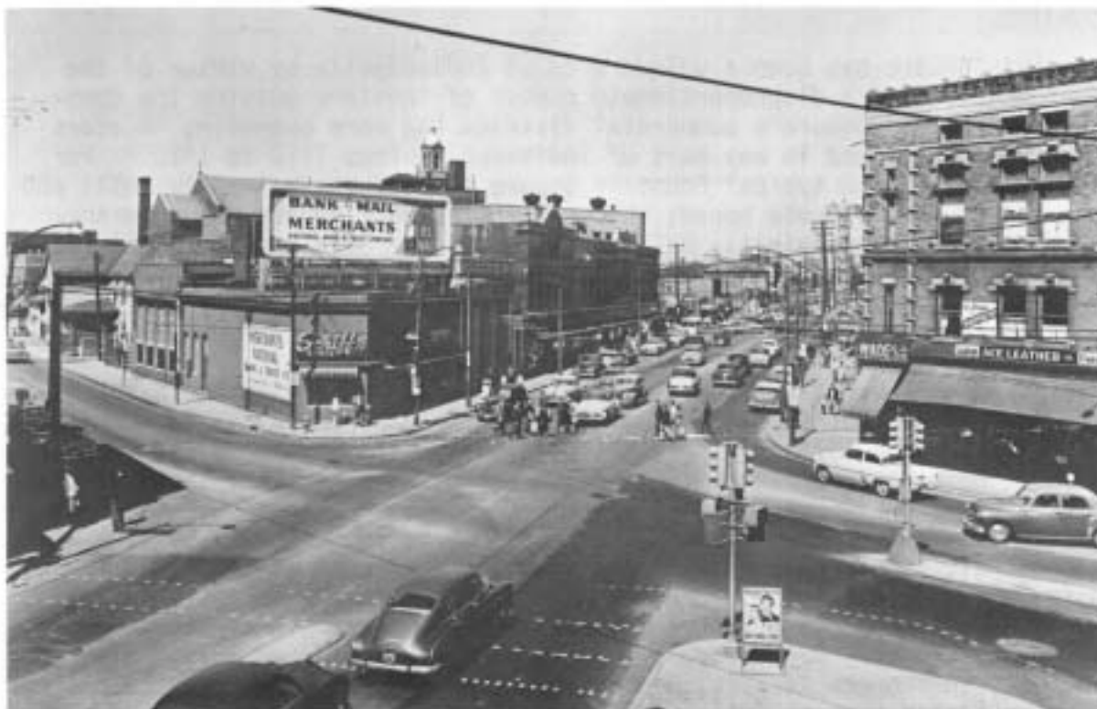
Virginia Avenue, looking northwest from Shelby Street, circa 1955, (top, Bass Photo Co.) and 1983 (bottom, IHPC Photo, ac).
