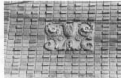
The brick work of a wall
